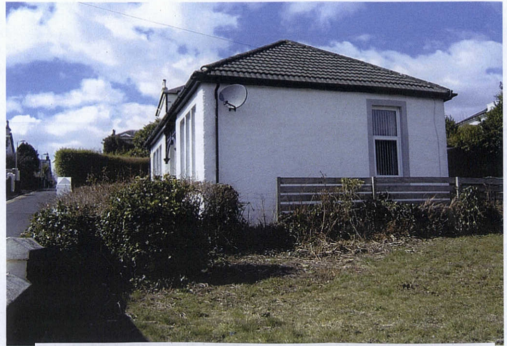
PROXIMITY TO BEDROOM WINDOW OF DWELLING AT 8 STEWART STREET
